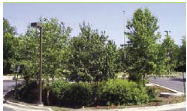
Infiltration planter/bioretention area
