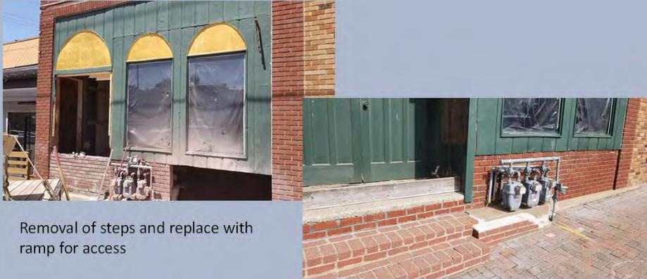
Removal of steps and replace with ramp for access
