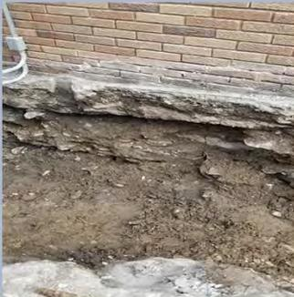
Waterproofing project uncovered defects in the foundation
