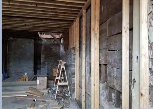
Reinforcement of exterior walls to support new replacement joists
