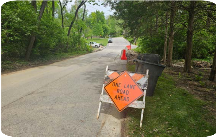
Elm St. is reduced to one lane due to stormwater damage
