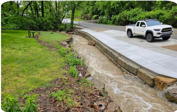
The new stormwater improvements on Crooked Rd in action
